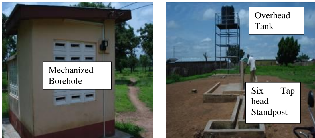
Picture 2: Borehole with Electric Pump, Overhead Tank and Standposts
