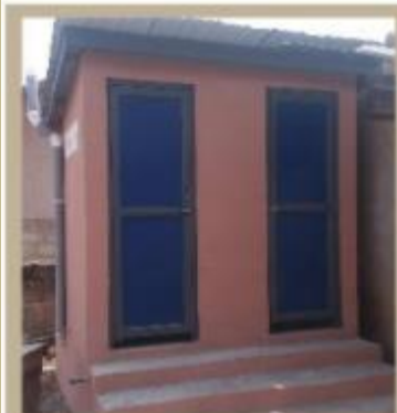
Stationary Block & Cement Toilet
