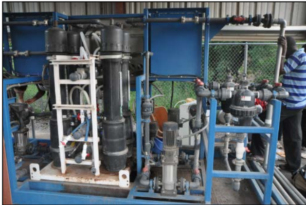
Manual controls replaced automated backwash so treatment can occur without electricity and repairs are easier. ( Technical Feasibility )
