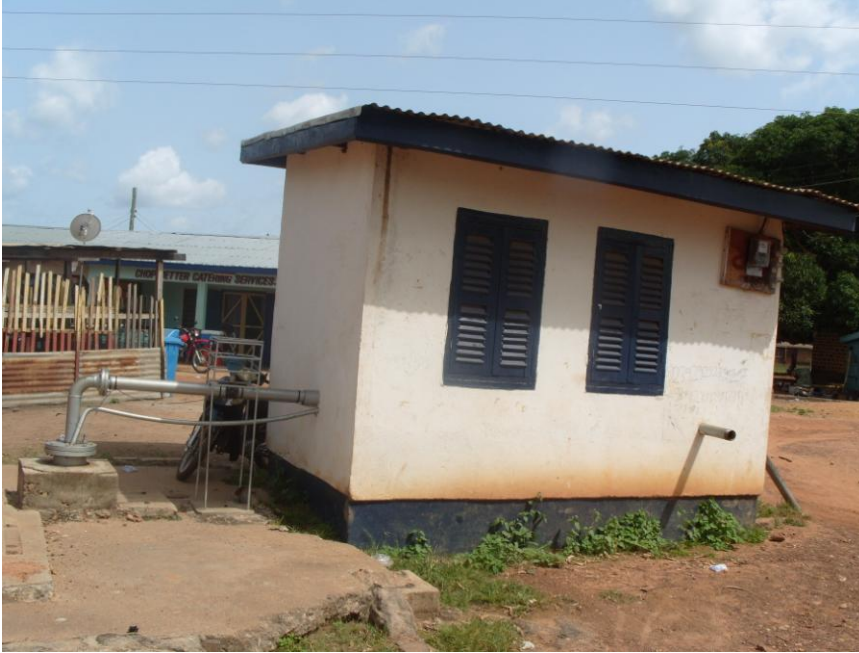
Picture 1: One of the Five Mechanized Boreholes of the Tumu Water System
