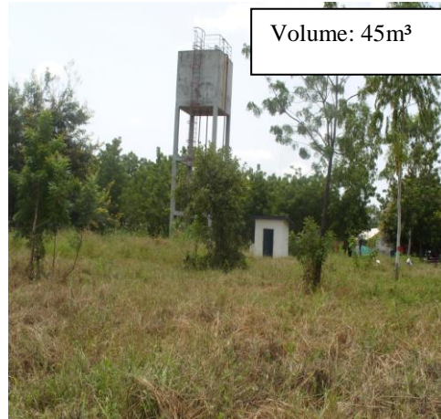
Picture 2: Elevated Tanks of the Tumu Water Supply System
