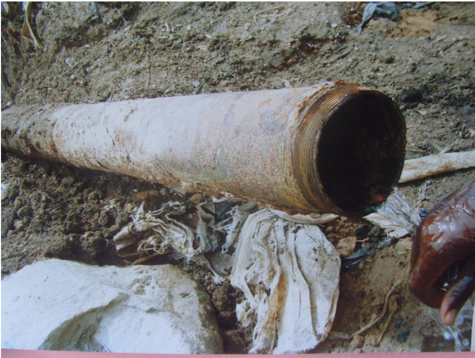
Picture 3: An Excavated worn Out Pipeline during System Maintenance
